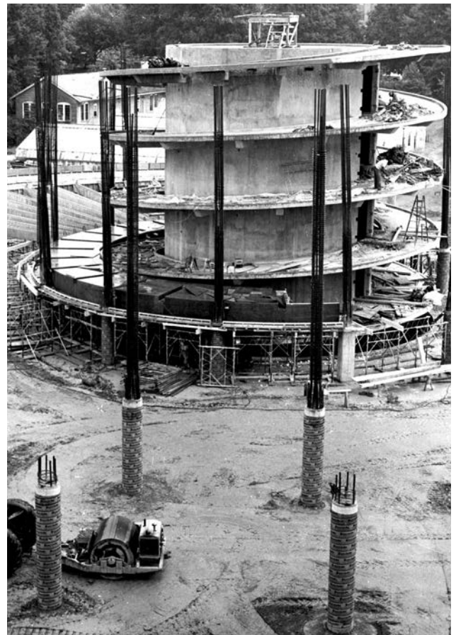
Construction of Harrelson's inner core. Photo by Ralph Mills.
